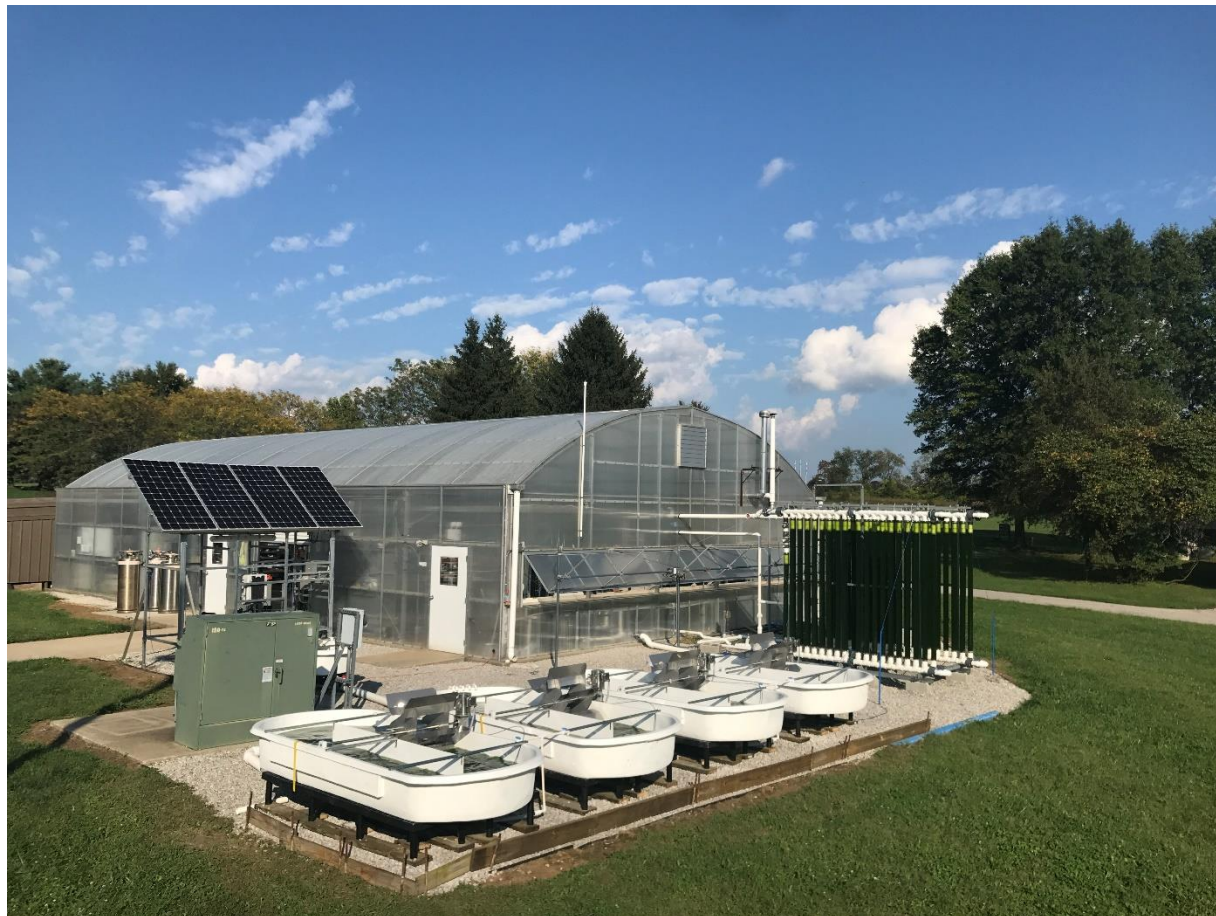
Ponds and cyclic flow PBR installed at UK CAER (10/6/2017)
