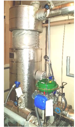
Single IDR installed at Canmet
