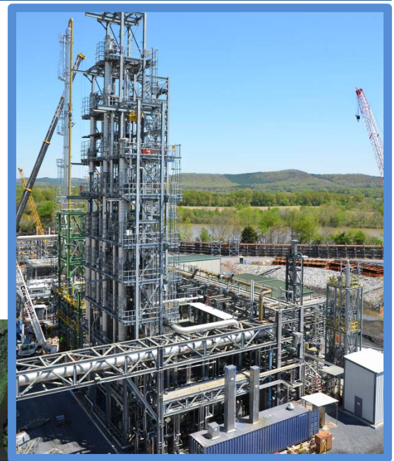
Post-Combustion Carbon Capture Center
