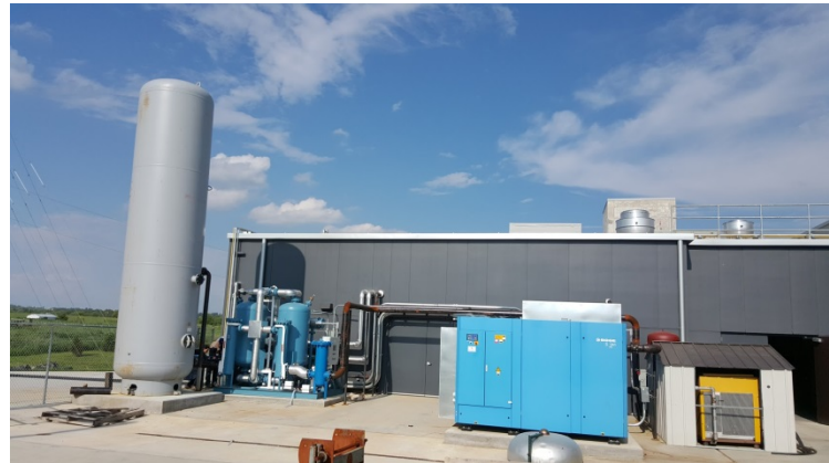
Rear View (from West)
