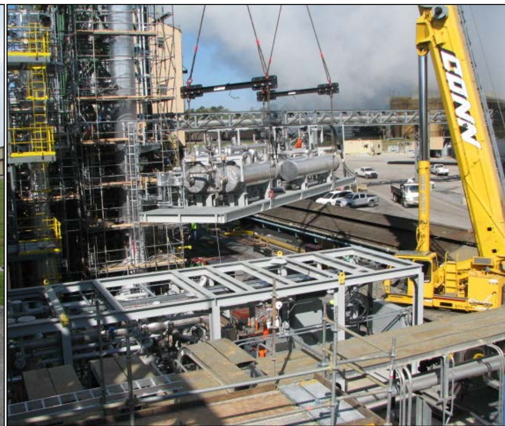
Crane lowering 2 nd floor of system into place
