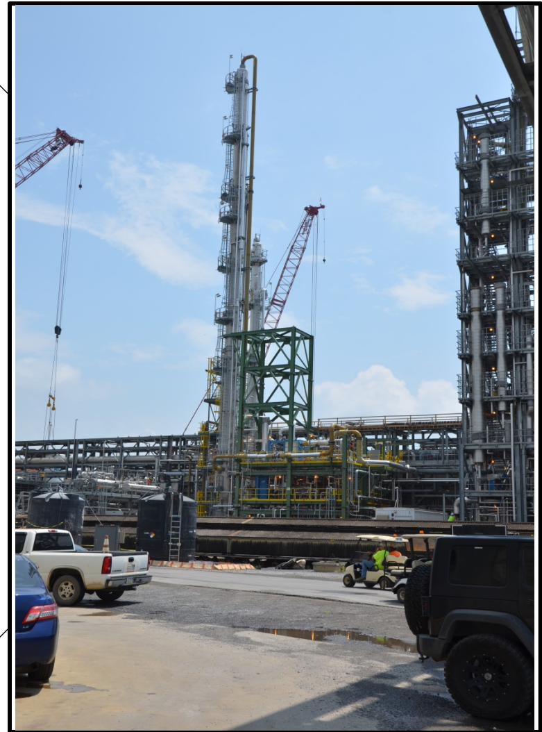
Linde-BASF 1 MW e pilot plant at the NCCC
