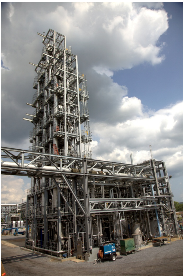
The NCCC PSTU
