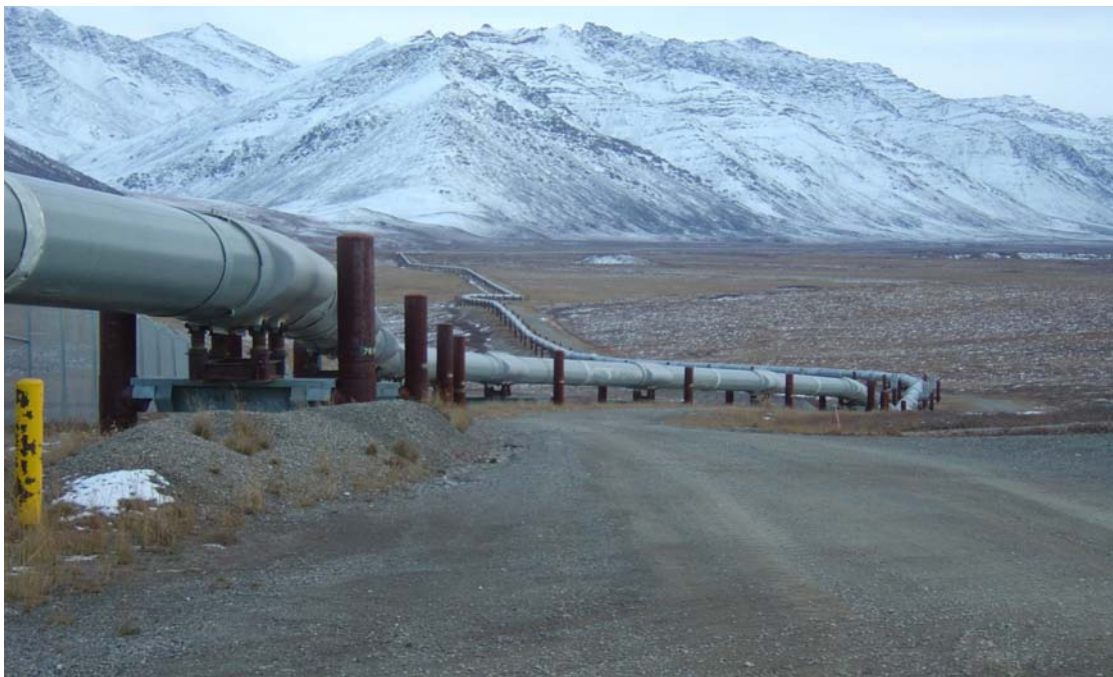
Trans Alaska Pipeline Traversing the Brooks Range
