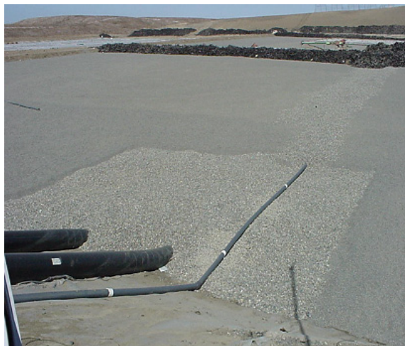
Waste Containment Base Liner System
