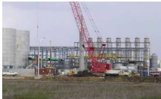
TAME Ethanol Plant Under Construction (Spring 2007), Greenville, Ohio
