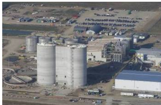
TAME Ethanol Plant about Two Months Prior to Startup (late 2007)
