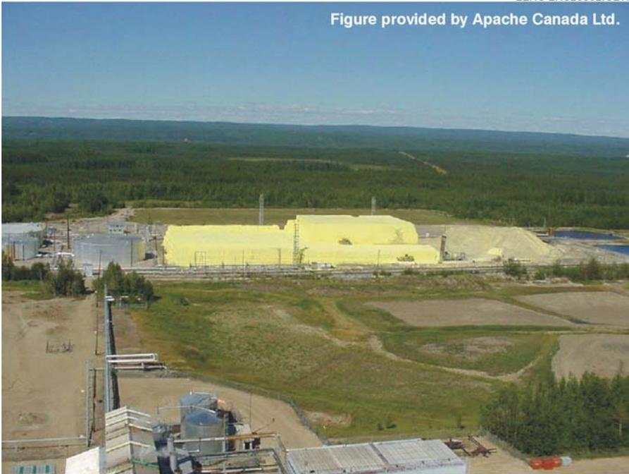
Figure 3. Elemental sulfur accumulating as a result of acid gas processing.
