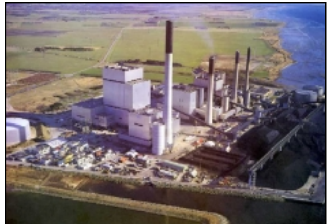
Figure 6b: ALSTOM Power Elsam project in Denmark (Nordjyllandsværket #3) (Net Oupput: 385 MW, Efficiency (LHV): 47%)
