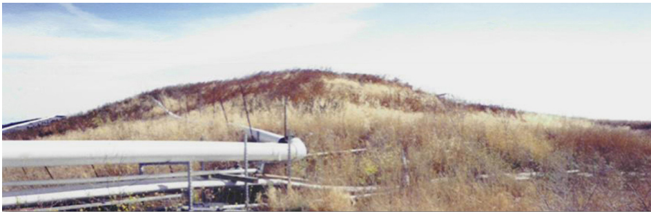
Figure 2 - Aerobic Cell at the Yolo County facility
