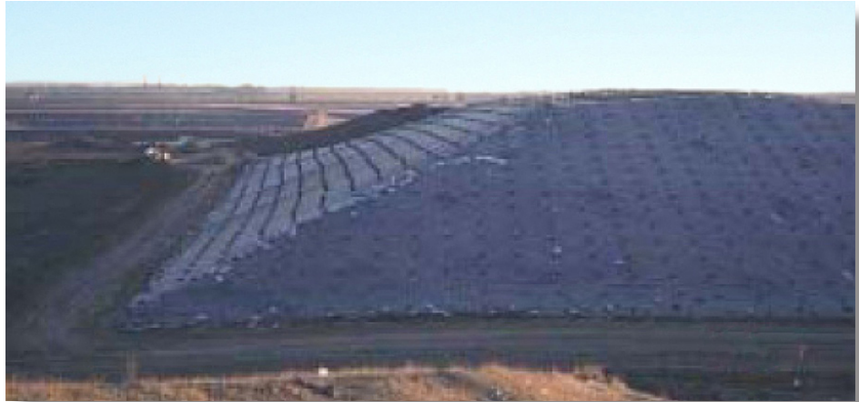
Figure 1 - Anaerobic Cell at the Yolo County facility
