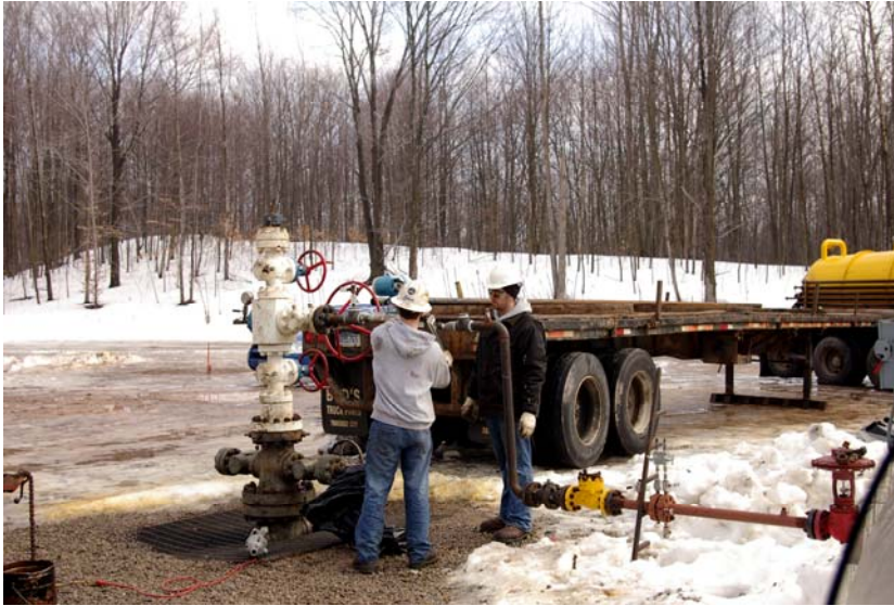
Figure 1. Preparing for CO 2 injection testing at the Otsego County, Michigan test site. Existing infrastructure was utilized for the field injection tests.
